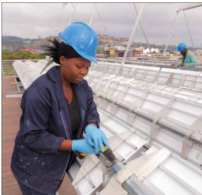
Montage der Anlage in Johannesburg – Installation of the system in Johannesburg
